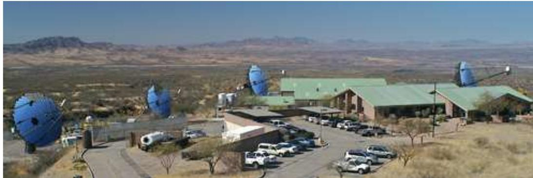
A rede de “telescópios” Čerenkov VERITAS (Very Energetic Radiation Imaging Telescope Array System) do Whipple observatory (Arizona), com quatro de  $D=12\text{m}$ . Detectam raios  $\gamma$  entre  $50\text{ GeV}$  e  $50\text{ TeV}$ .
